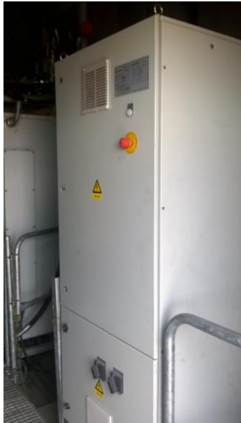
Armario Ground Controller, sin pantalla de control. Ground controller cabinet, without control screen
